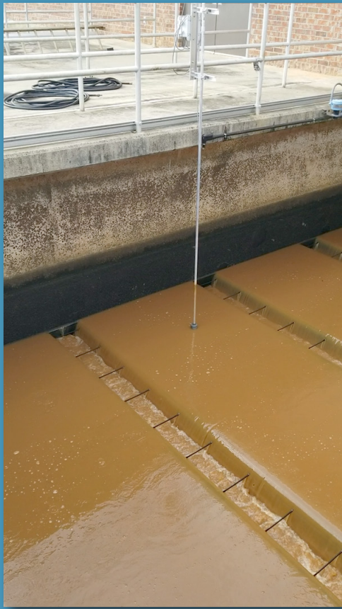
A full mud boil at the height of a high wash
